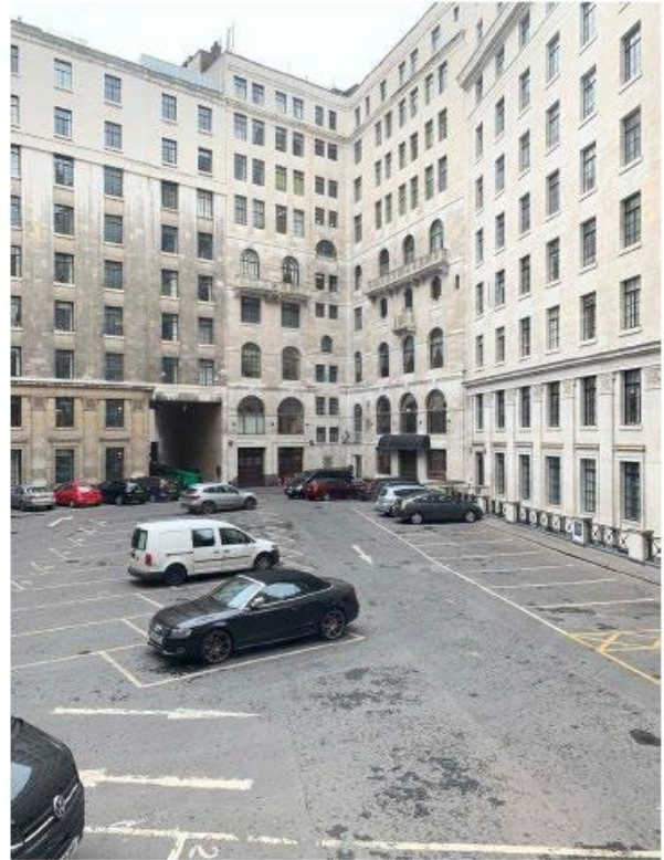
Courtyard Elevations of Surrounding Buildings
